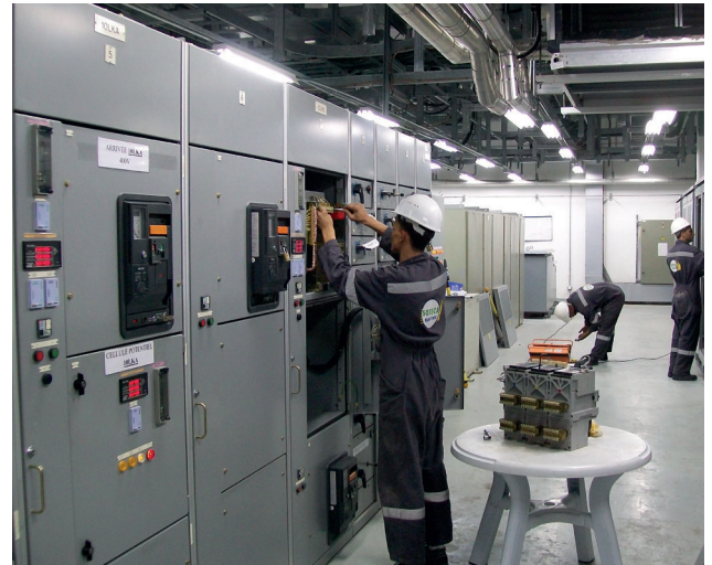
Project: Electrical Maintenance for withdrawable cabinets for a power plant (Terga - Algeria) Year: 2014
