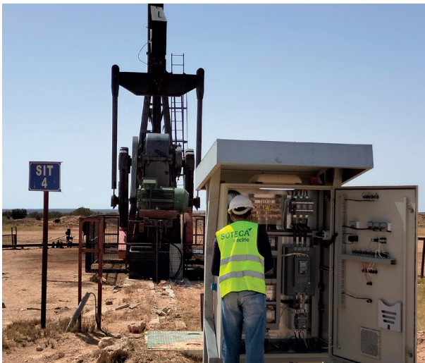
Project: Electrical Installation (Bir Mellouli - Tunisia) Year: 2021
