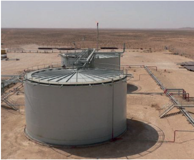
Project: Maintenance of electrical panels at the production stations in Kerkennah & Matmata (Tunisia) Year: 2010
