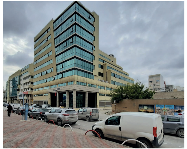
Project: African Development Bank (Tunis - Tunisia) Client: African Development Bank
