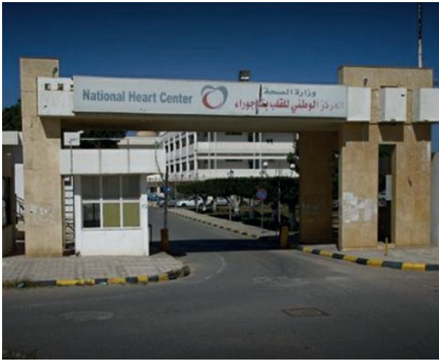
Project: Electrical panels (Tajoura, Tripoli - Libya) Client: National Heart Center Hospital
