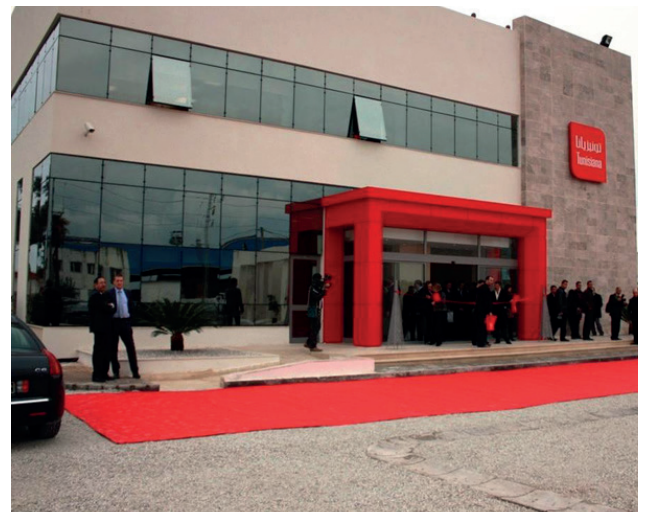
Project: Electrical installation for all of Ooredoo's shops (Tunisia) Client: Ooredoo
