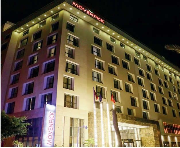
Project: Mövenpick Hotel (Sfax - Tunisia) Client: Mövenpick Hotels & Resorts
