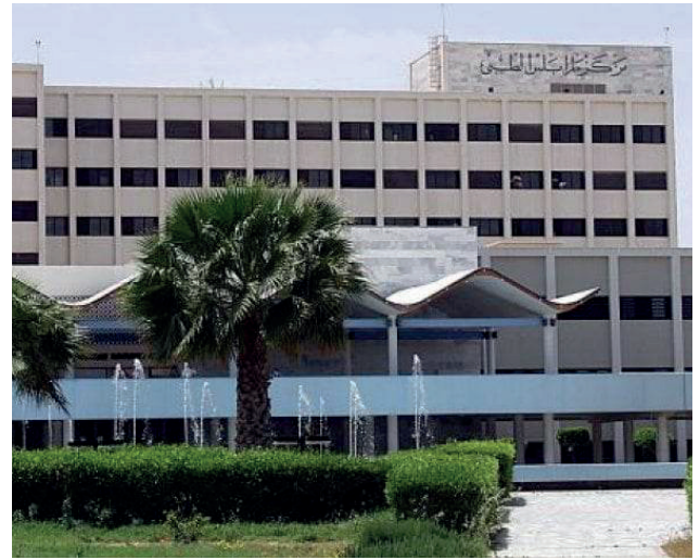
Project: Electrical Maintenance (Espiaa, Tripoli - Libya) Client: Tripoli medical center
