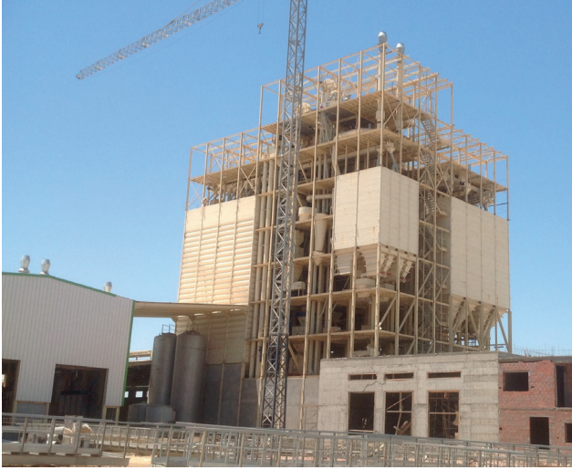
Project: Cattle Feed Factory (Tunisia) Client: Medimix
