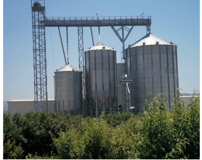
Project: Cattle Feed Factory (Algeria) Client: Khnis
