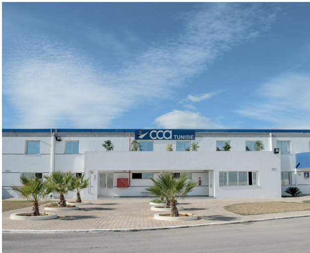
Project: Electrical Installations (Tunis - Tunisia)
