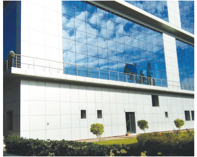
Project: Electrical installation (Algeria) Client: Industries Médico-Chirurgicales (IMC)
