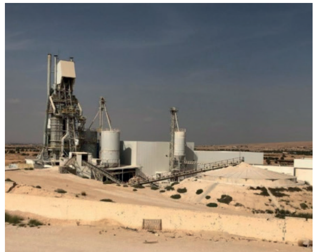
Project: Electrical installations (Gabes - Tunisia) Client: Carmeuse
