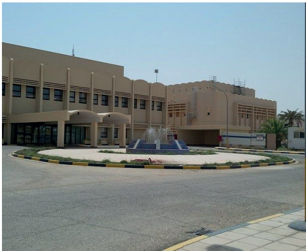
Project: Electrical installation (Al Kassim - Saudi Arabia) Client: Spimaco
