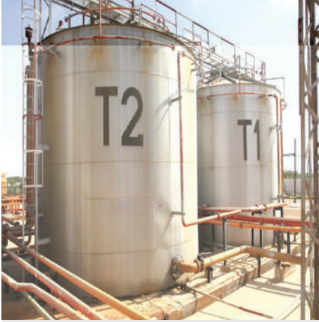
Project: Electrical works (Tunisia) Client: CTKCP
