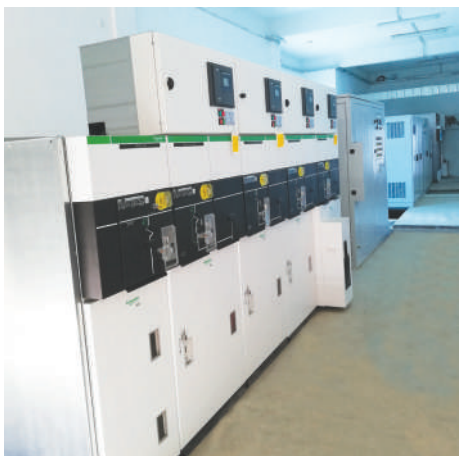
Project: Fuel Storage Center - Sidi Bel Abbes (Algeria) Scope: Supply & Installation of MV Substation Client: SONATRACH
